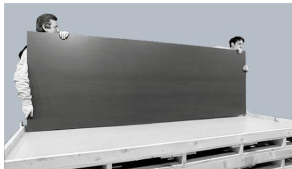
2 | Guide the slab to its upright position, keeping it as straight as possible.
